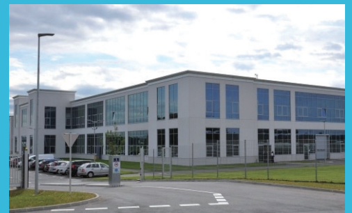
MSBS(Magna Steyr Battery Systems)
