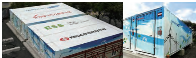
Jocheon Substation in Jeju, Korea (8MWh)
