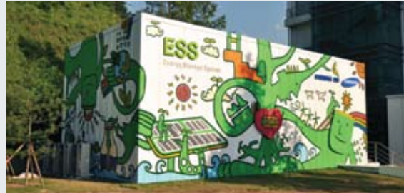
1MWh scale ESS at Samsung SDI Giheung Plant
