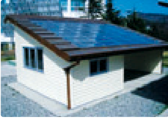
First Polycrystalline Si PV House: 3kW PV System
